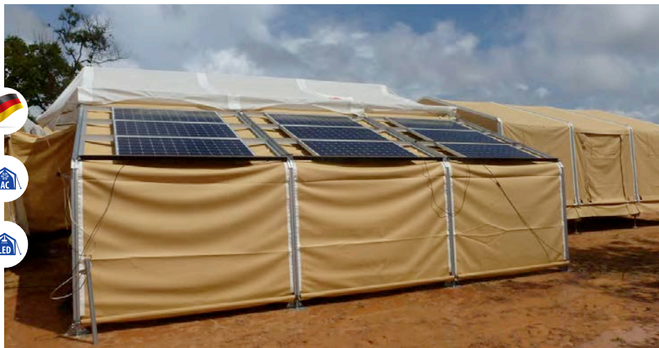
Schall: Alu-framed highly insulated tent with solar power panels providing shelter for the fuel laboratory at the Bulk Fuel Installation. Connected to the micro grid using the PFISTERER MEMS.
