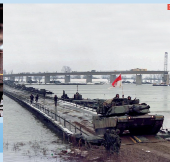
3 The pontoon bridge erected over the Sava River by the US Army's 1st Armored Division, allowing IFOR troops to cross from Croatia into Bosnia and Herzegovina.
