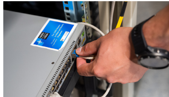
Figure 6. Detail of the Quantum Key Distribution setup at the Faculty of Electrical Engineering and Computer Science of the Technical University of Ostrava, Czech Republic.
