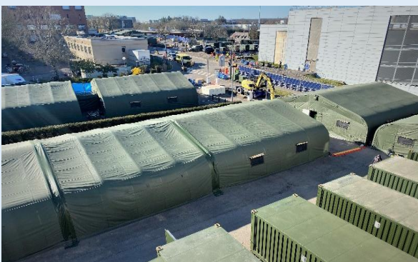
Field hospital built at Centre Hospitalier du Luxembourg
