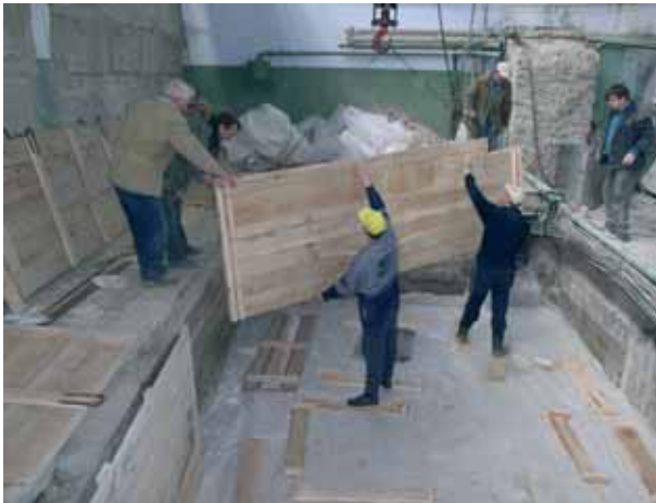
A basement is built to house the cyclotron x-ray device
