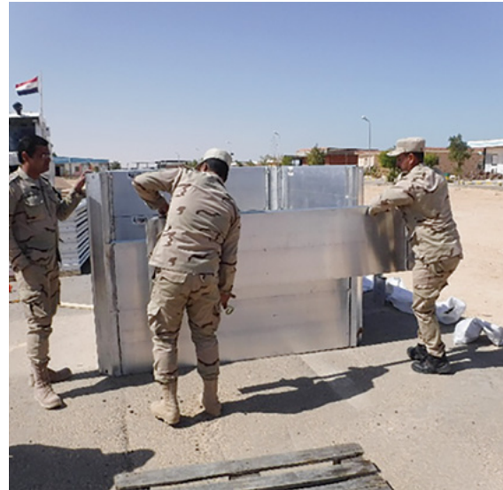
Figure 10 – Demonstration of usage of shoring box panels during C-IED training for the Egyptian Corps of Engineers.
